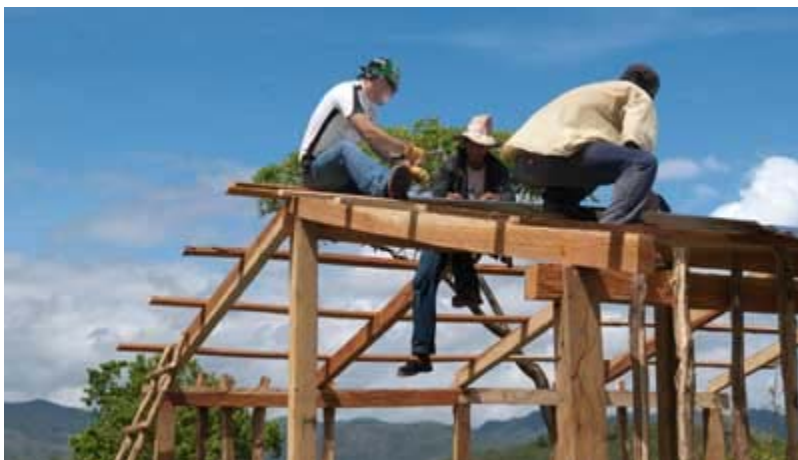
Austin on a roof helping build a new home
